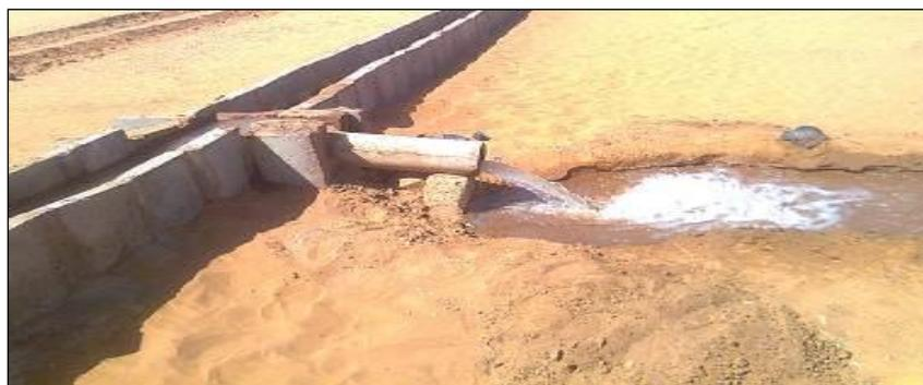
**Plate 3. A lined section and field out-let pipe made of local aggregates**
