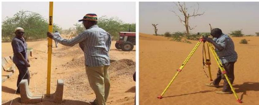
**Plate 2. Set out of the hydraulic slope and channel alignment**
