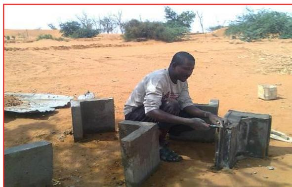
**Plate 1. Precasing and release of the form**
